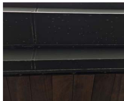
Examples of salt deposits on soffits and undersides of gutters
