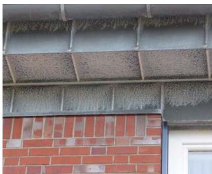
Examples of salt deposits on soffits and undersides of gutters
